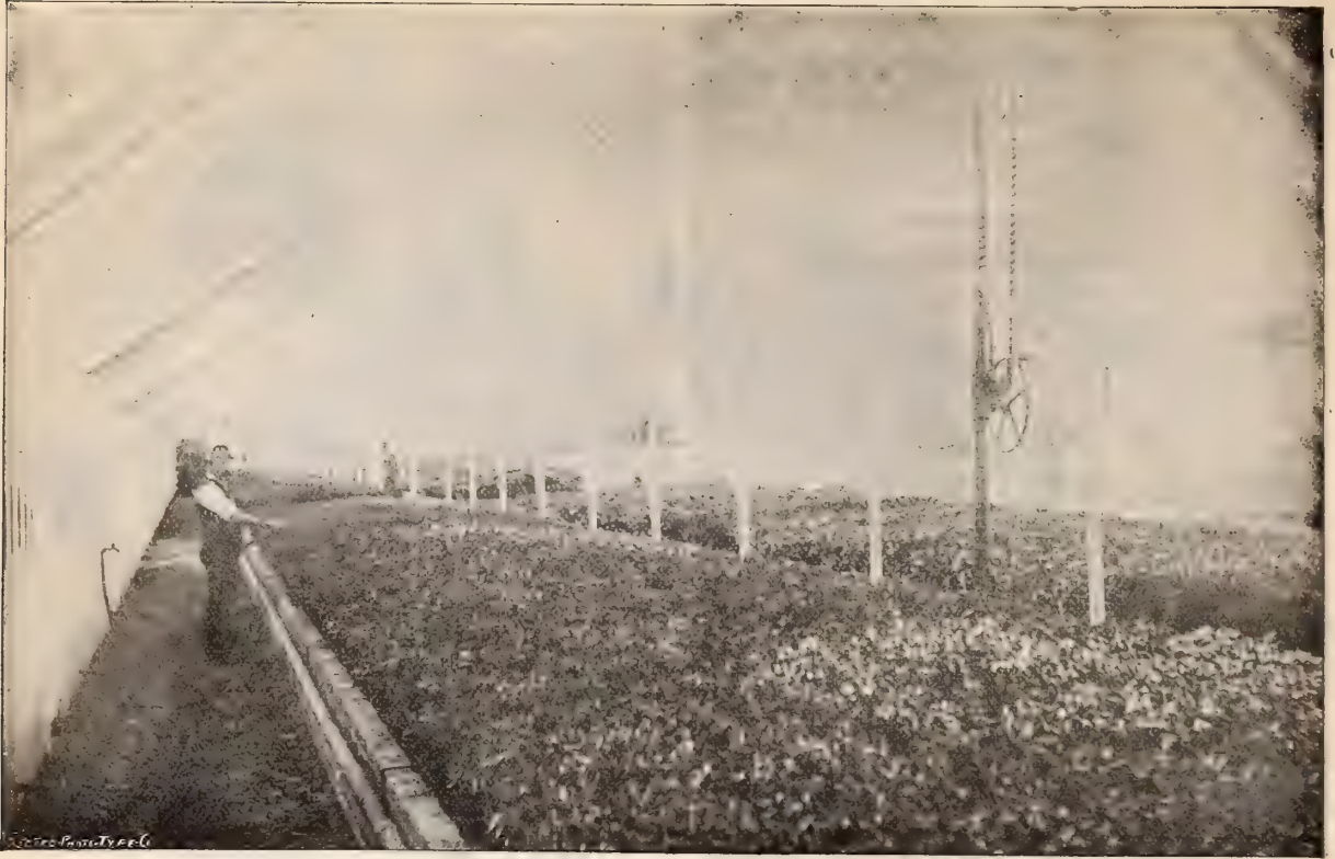
VIEW OF HOUSE OF AZALEAS, 252 X 25 FEET.—From a photograph.
